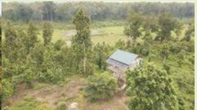
Aerial view of community watch tower
